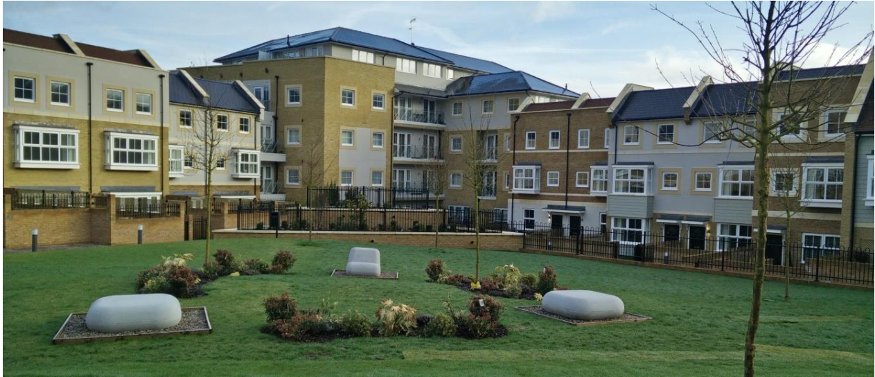
Figure 1. View of the development from the courtyard.
